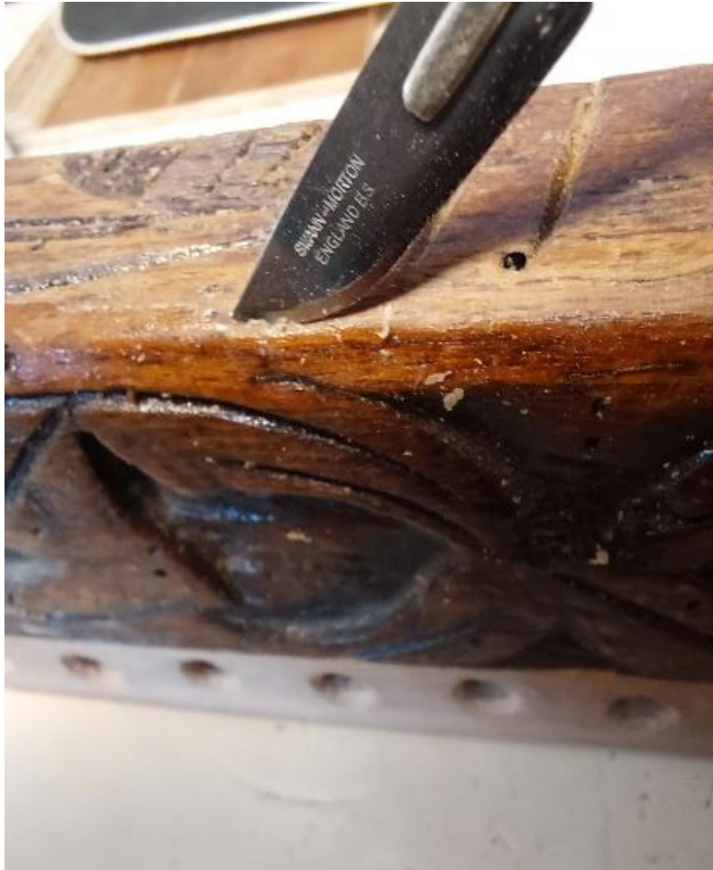
Fig 5, Scraping off the surface, the hardened consolidator off
